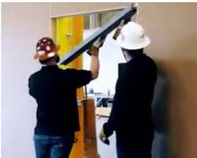
4. Slip the frame head over the rough opening header and center it in the opening.
