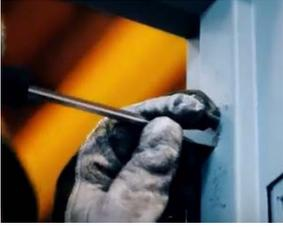
8. Snug the compression anchors evenly in each jamb. Use a level and a framing square to check for plumb, square, and twist.
