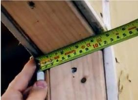
3. Measure the thickness of the wall for the frame throat opening. Be sure to check where the vertical studs meet the header.
