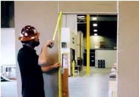
2. Measure the width and height of the rough opening to ensure they meet the manufacturer's recommendations.
