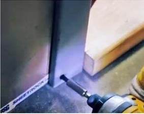
9. Anchor the base of the hinge jamb to both faces of the wall using the provided anchor system. Repeat the process for the strike jamb and remove the spreader bar when installation is complete.
