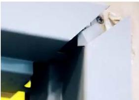
5. Install the hinge jamb by slipping it over the wall at an angle and engaging the jamb into the head. Finish straightening the jamb by slipping it over the wall, ensuring the drywall has entered the frame throat opening on both faces of the wall.
